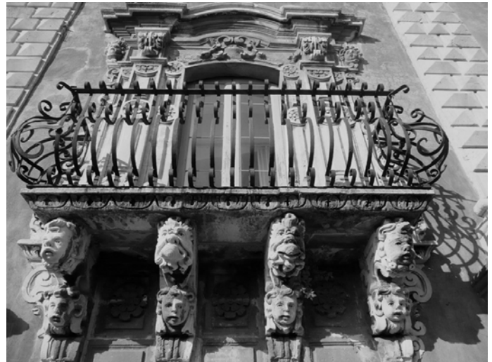
A balcony on the Monastery of Saint Nicholas in Catania, showing the mascheroni, or mask-like decoration, and wrought-iron balconies, variations of which are common in Sicily. The use of grey and white stone and the rusticated pilasters on either side of the balcony are more typical of the Catania area.
