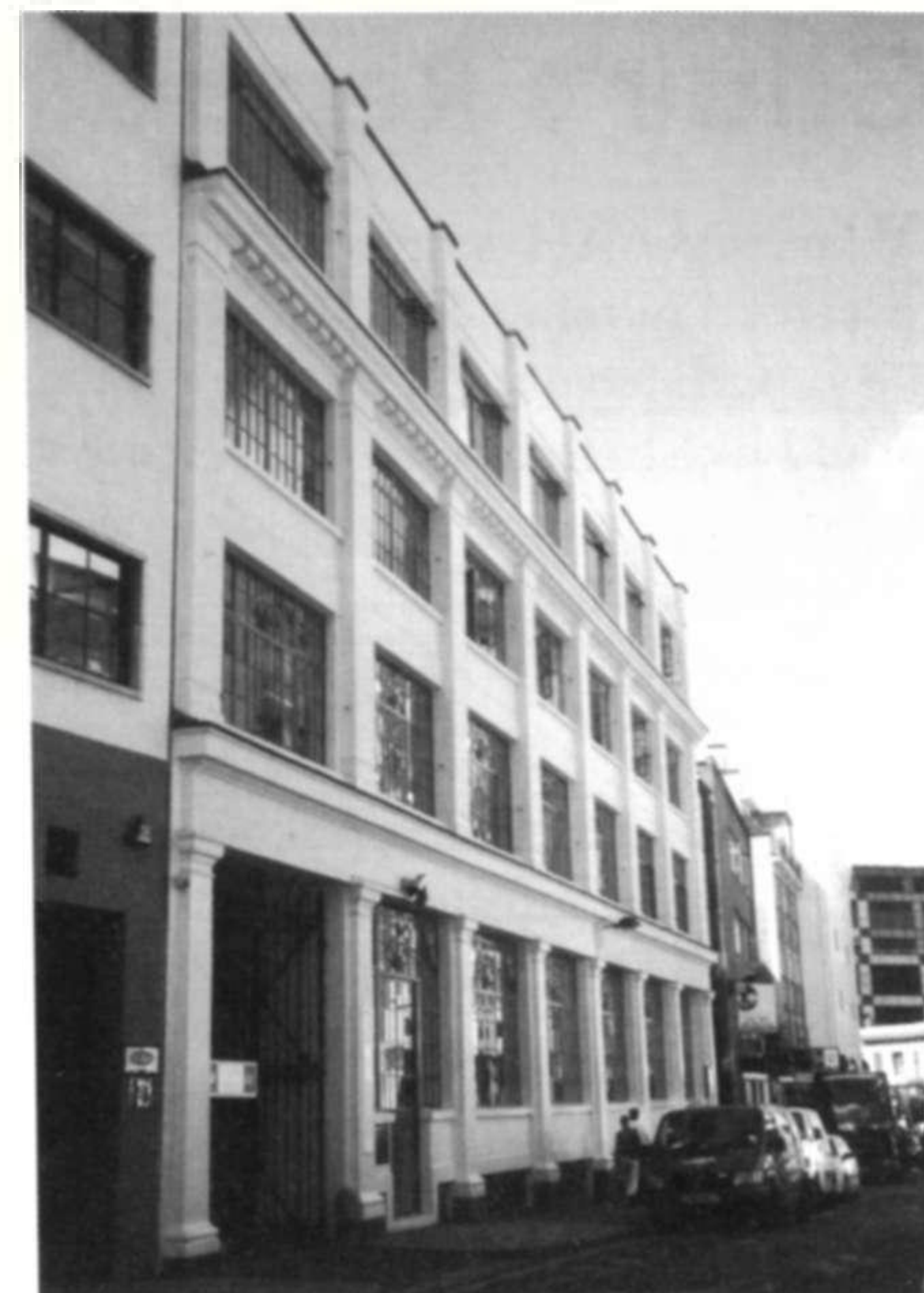
A view from the street of Cowcross Court
